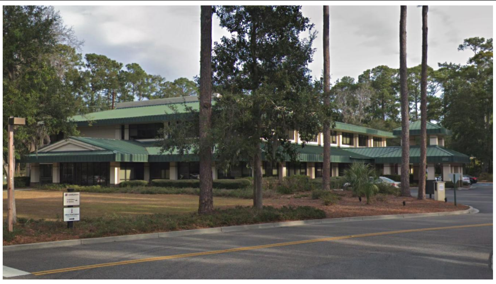
ADJACENT BUILDING - 870 W.M. HILTON PARKWAY
