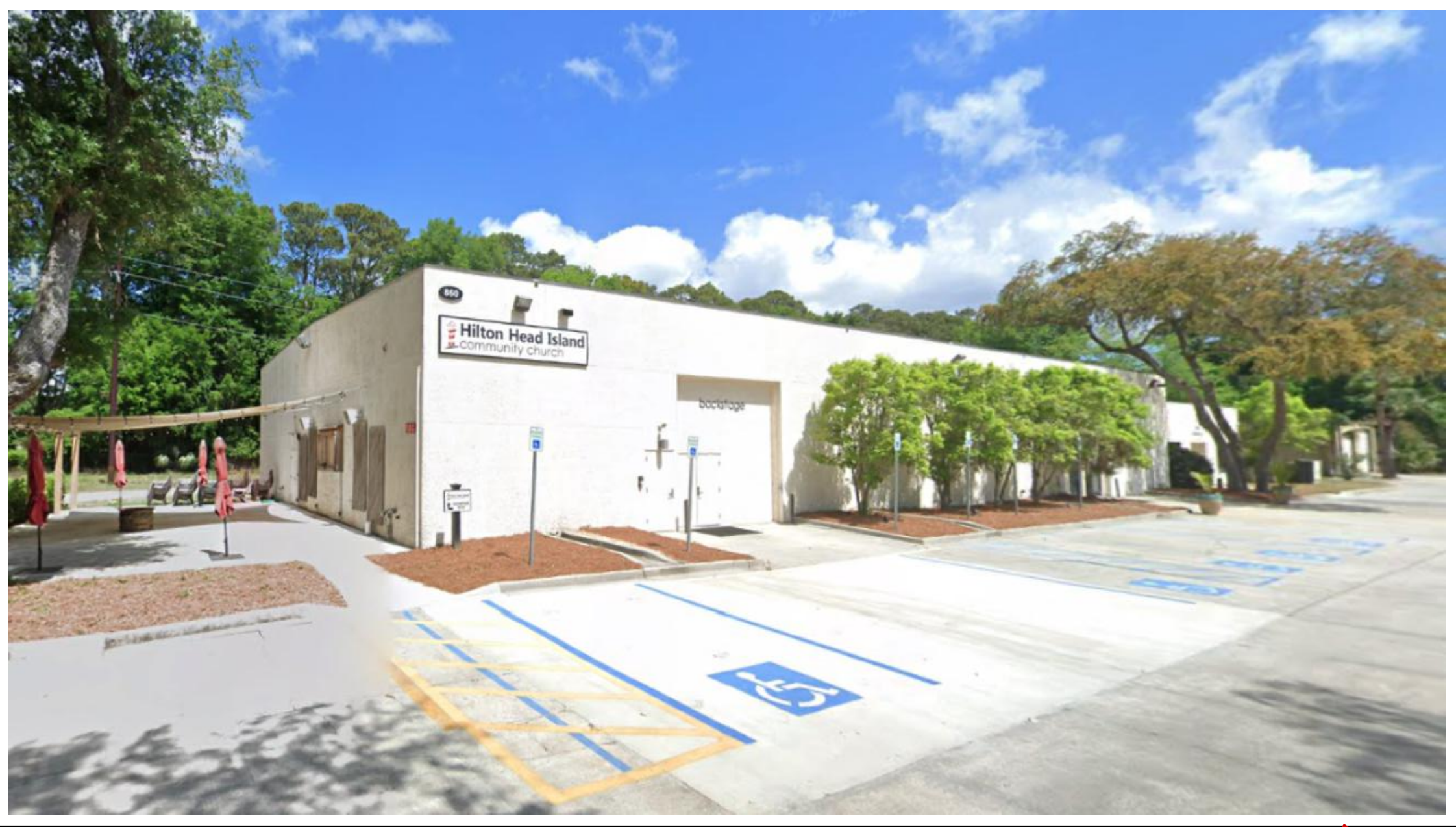
ADJACENT CHURCH UTILITY BUILDING - 860B W.M. HILTON PARKWAY
