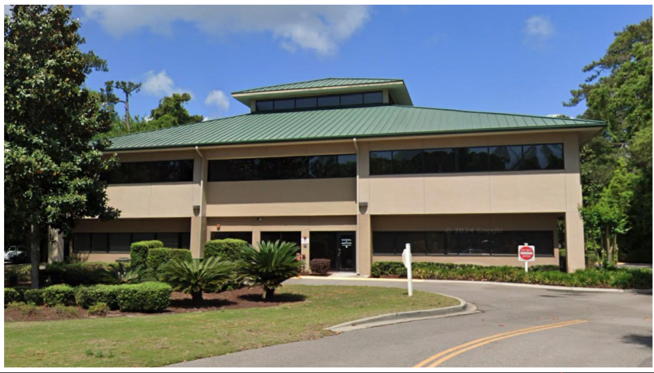
COLLINS REALTY BUILDING - 852 W.M. HILTON PARKWAY
