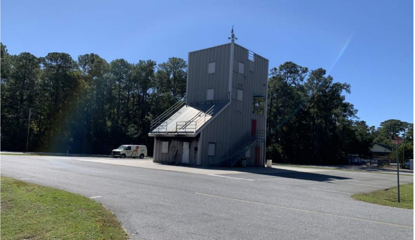
View of training tower taken from adjacent to project site.
