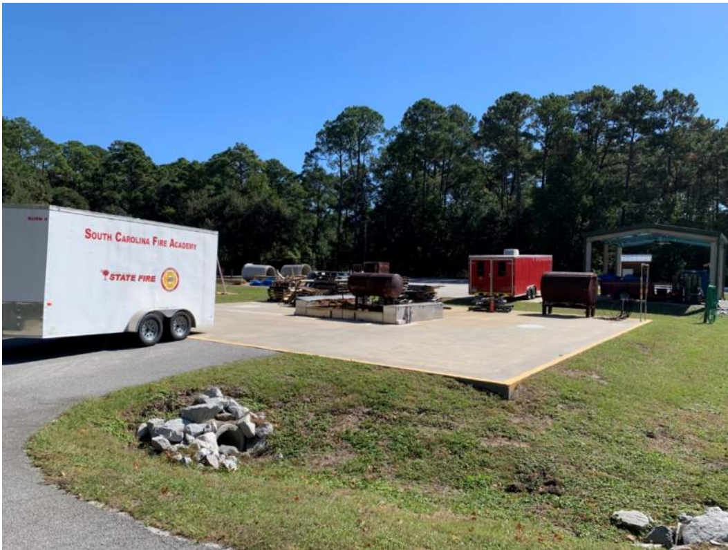
View of existing concrete pad where building will be located.
