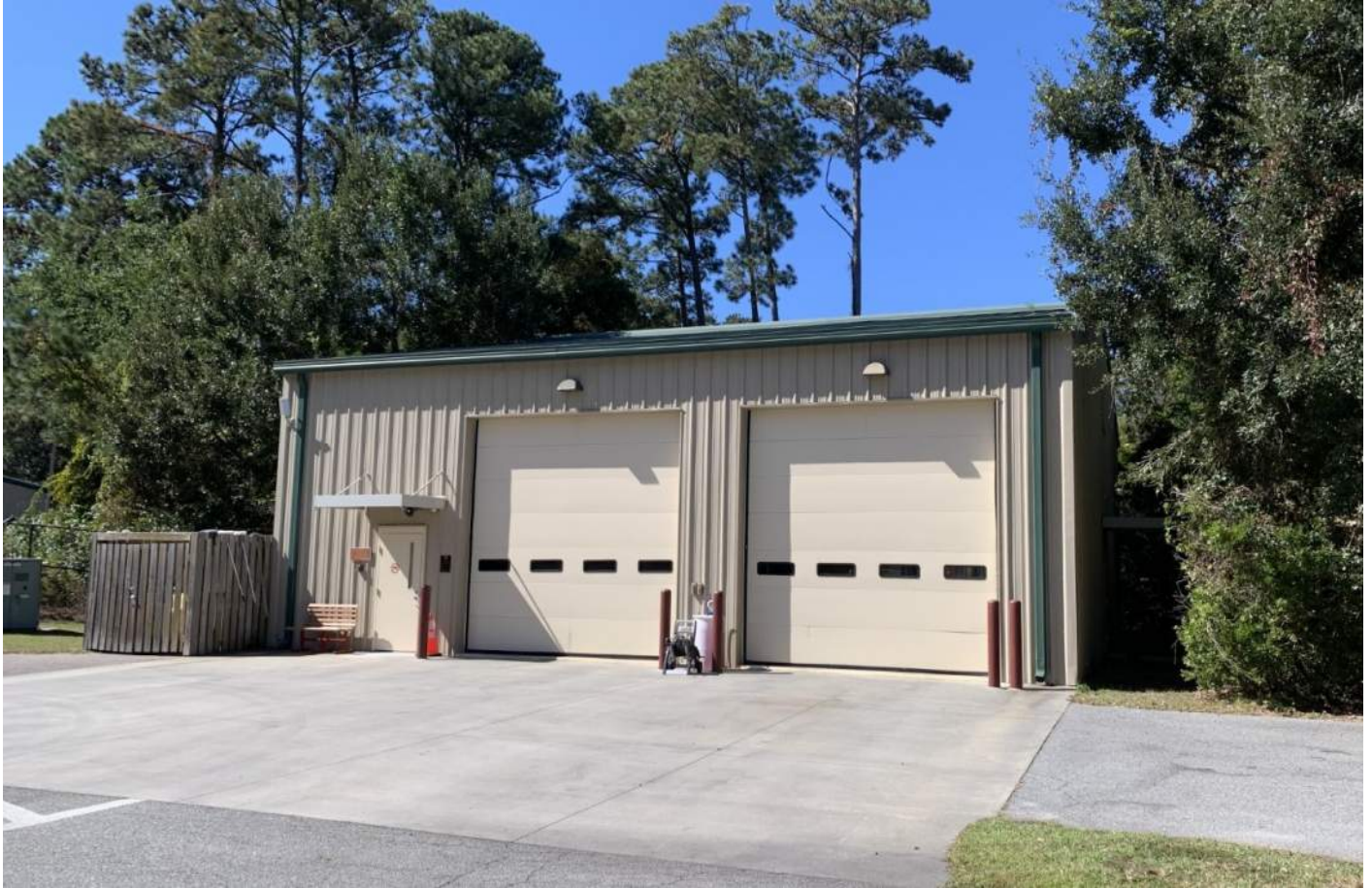
View of pre-engineered storage building.
