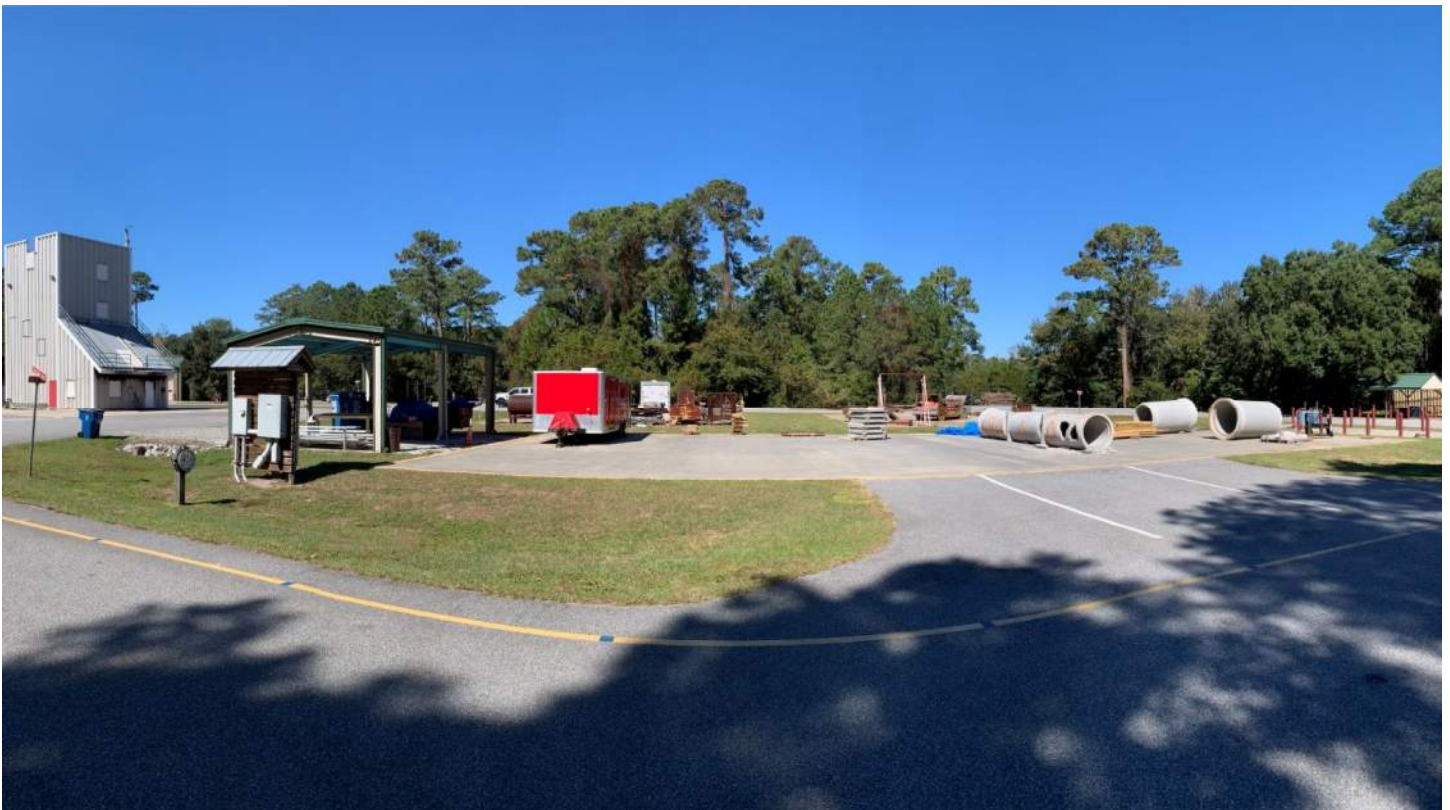
View of extrication pad in foreground, covered building at left. Project site located behind red trailer.
