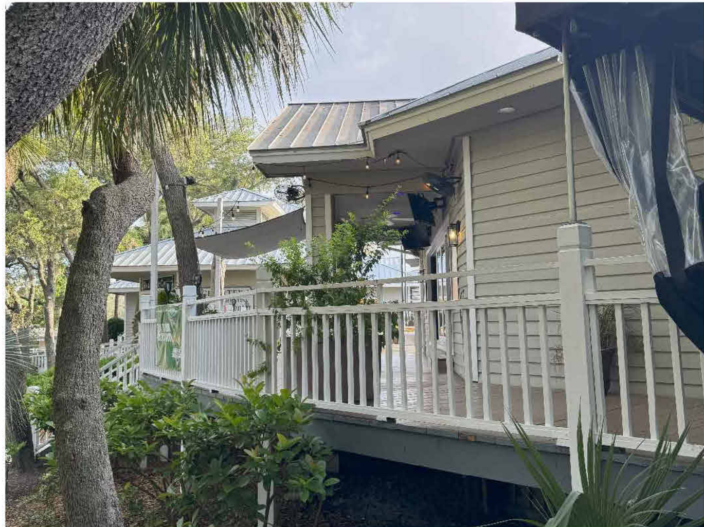
7: RIGHT SIDE OF DECK W/ FABRIC ROOF AREA TO RIGHT
