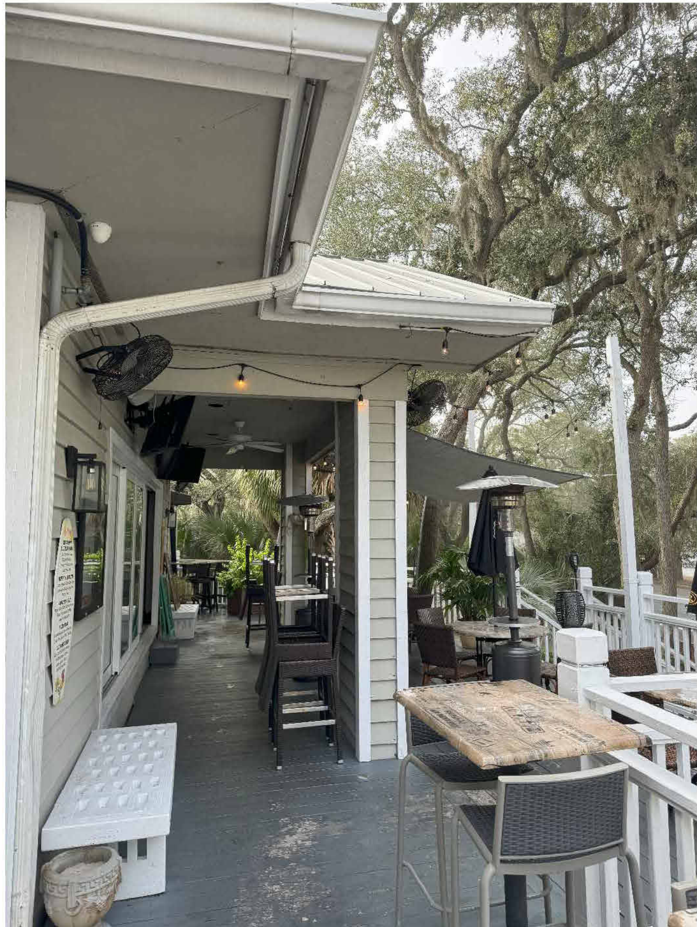
4: DECK AREA TO BE COVERED & LEFT SIDE OF FRONT PORCH
