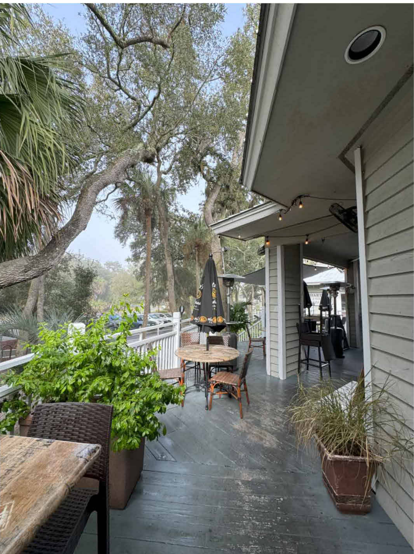
6: DECK AREA TO BE COVERED & RIGHT SIDE OF FRONT PORCH
