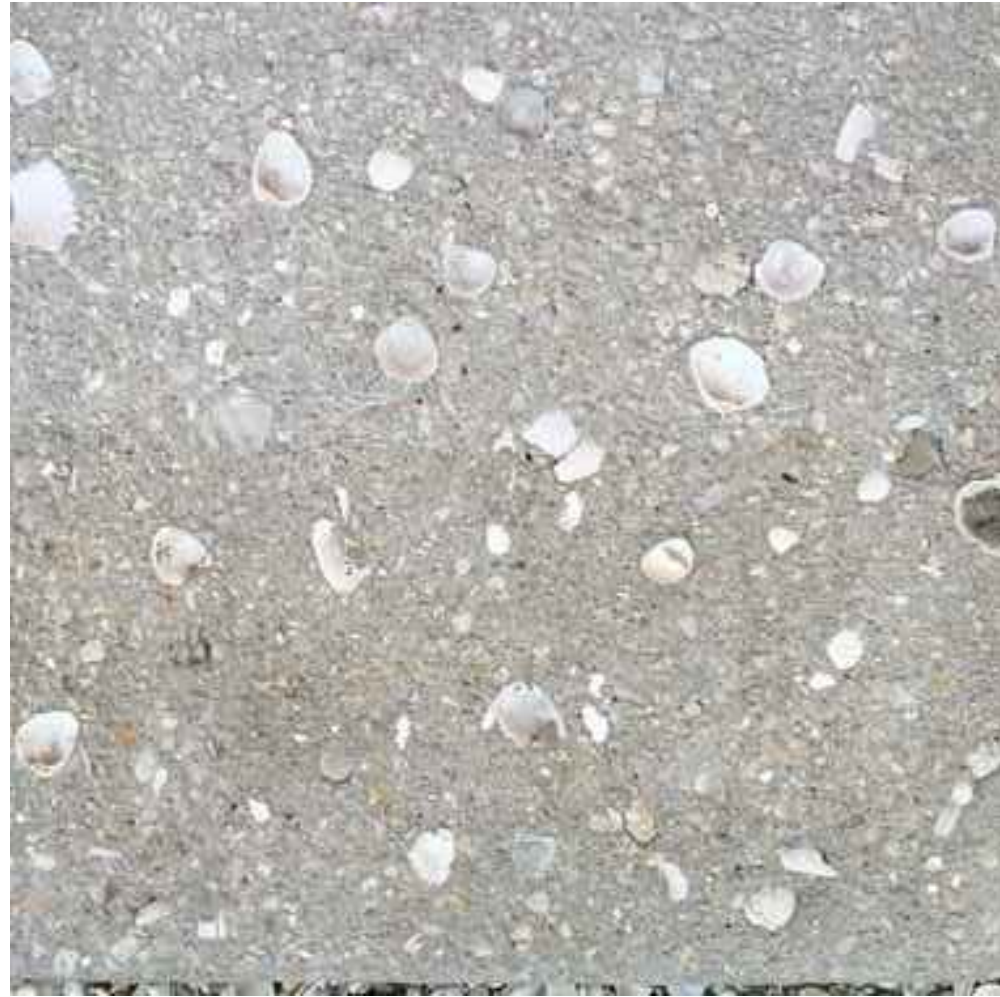
1 PAVEMENT TYPE 1 (OYSTER SHELL CONCRETE)
