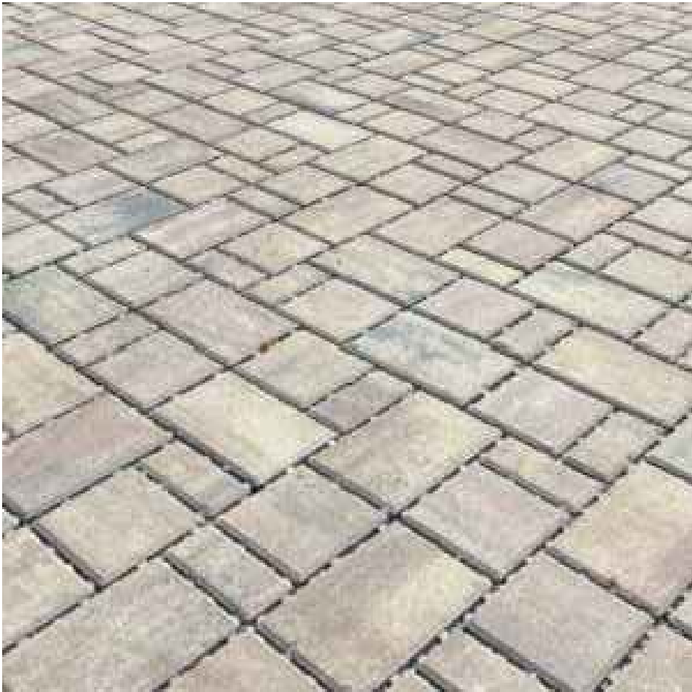
3 PAVEMENT TYPE 3 (PERMEABLE PAVER - 3-PIECE)
