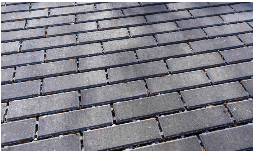
2 PAVEMENT TYPE 2 (PERMEABLE PAVER - LINEAR)
