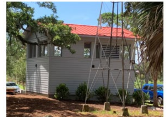
Lawton Control Building
