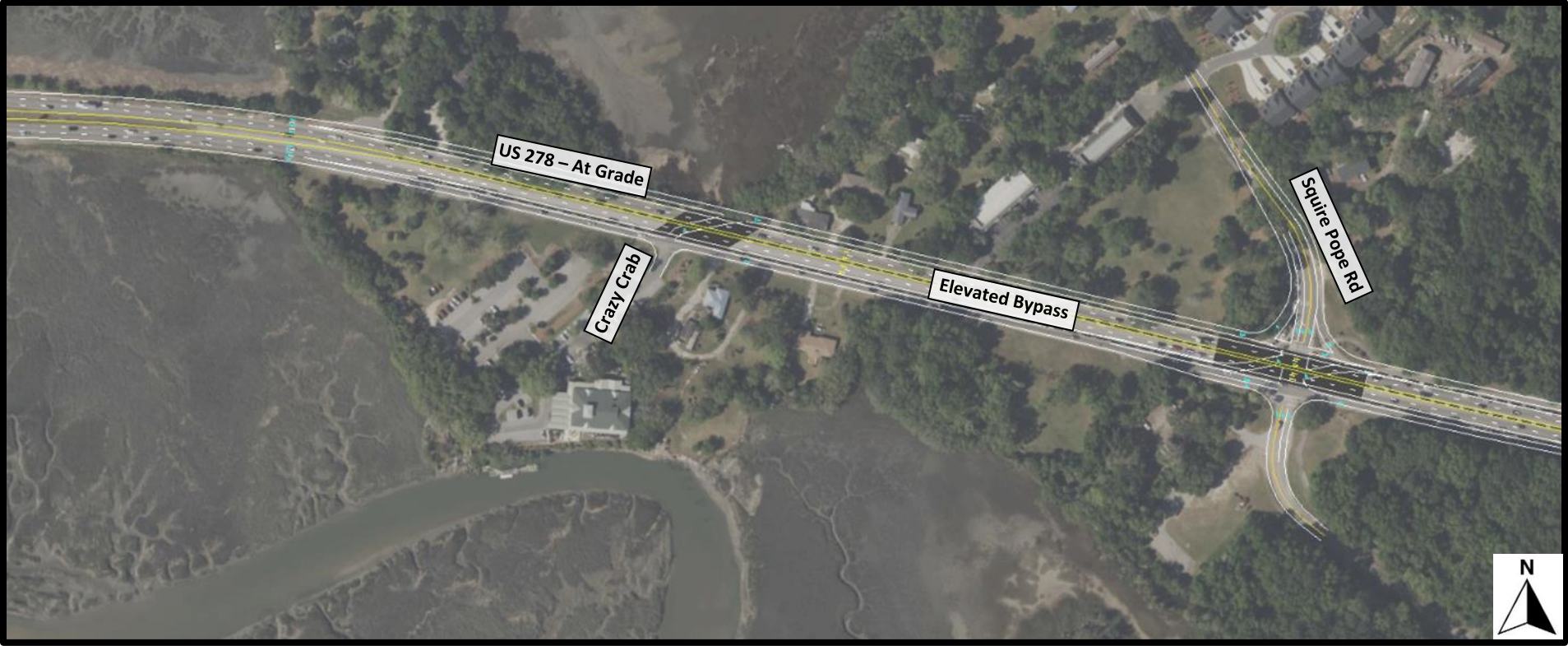
Figure 7. Example of Elevated Bypass - 01
