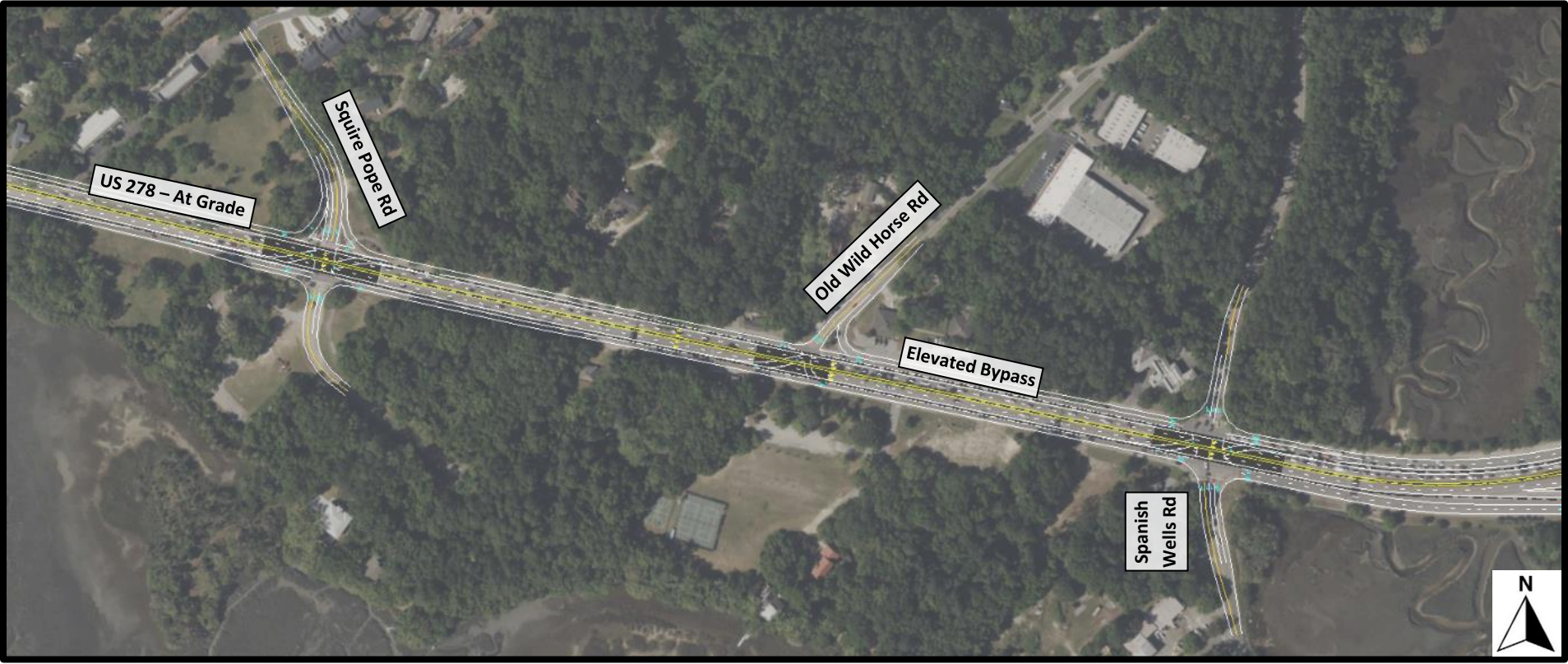
Figure 8. Example of Elevated Bypass - 02
