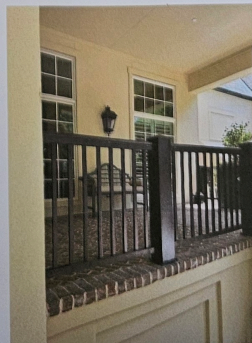
7 & 8 – DOOR HARDWARE & HANDRAILS
