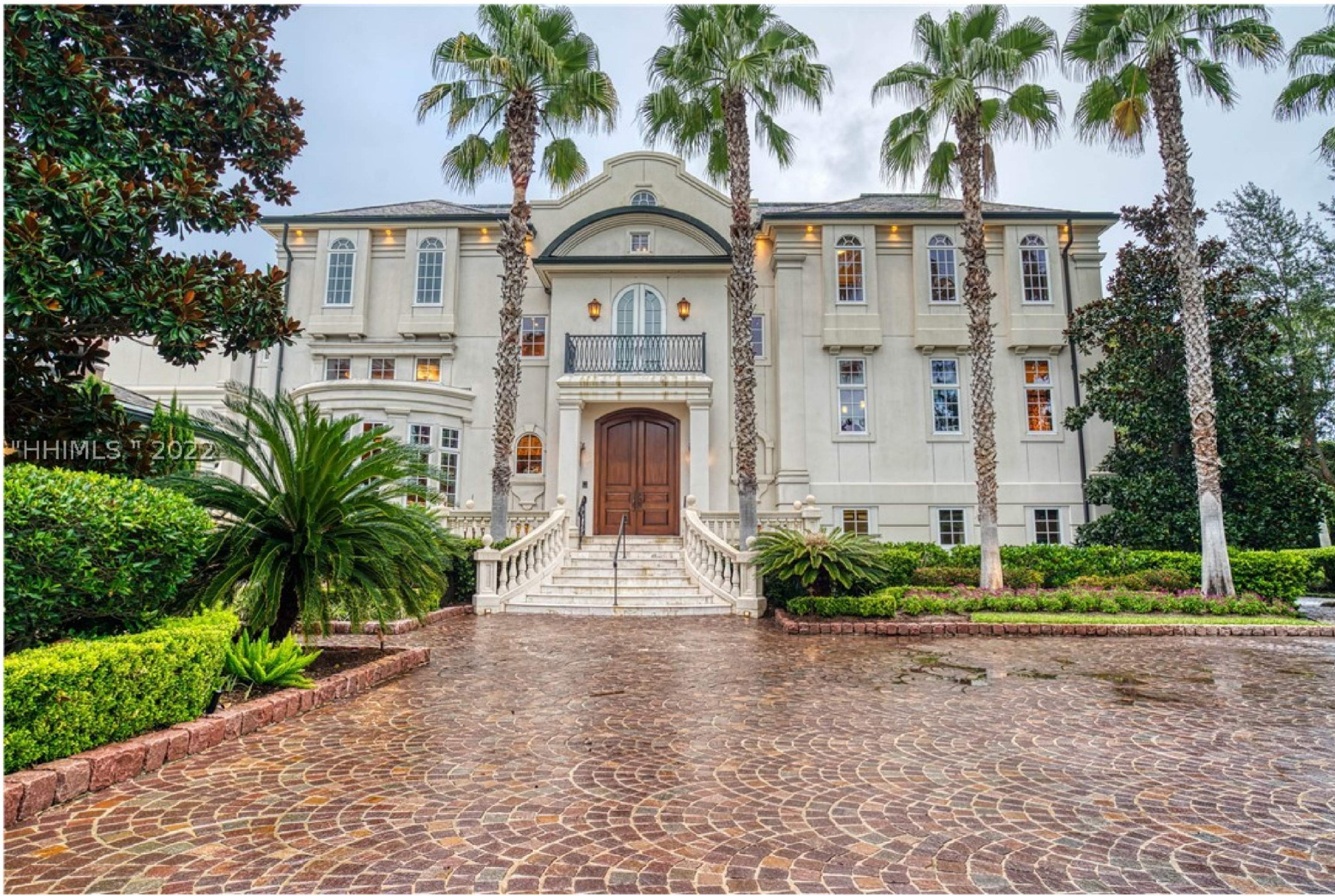
NEARBY RESIDENTIAL PROPERTY (80 BRIDGETOWN LANE)
