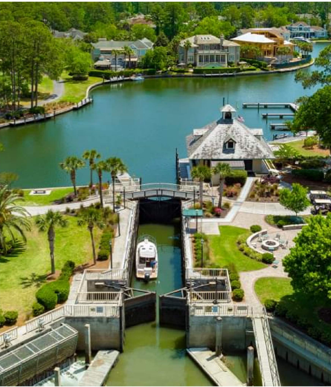
EXISTING WEXFORD HARBOUR MASTER BUILDING
