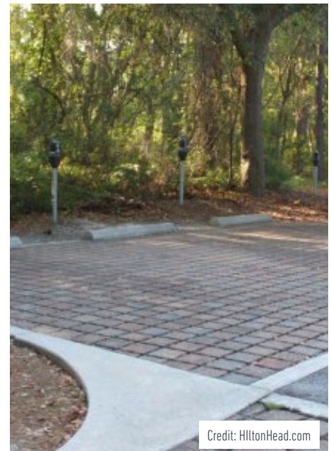
Pervious parking areas, like the system picture above at Islanders Beach Park, allow rain water to percolate into the ground. This helps to re-charge ground water aquifers and minimize run-off.
