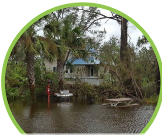
Damage from the 2016 storm Hurricane Matthew. Credit: Island Club of Hilton Head
