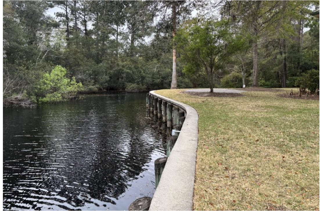
7 LAGOON BULKHEAD WALL
