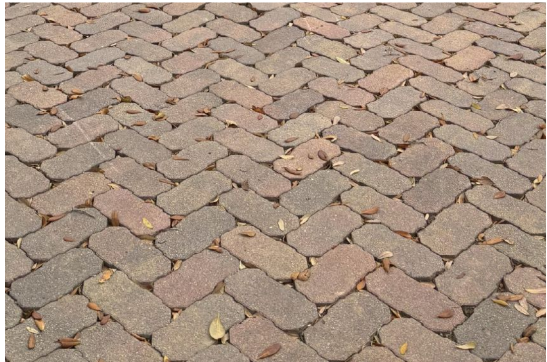
9 PERVIOUS PARKING SURFACE
