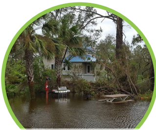
Damage from the 2016 storm Hurricane Matthew. Credit: Island Club of Hilton Head
