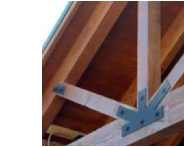
MED. WOOD FINISH TRUSS W/ BRONZE PAINT MATCHED TRUSS BRACKETS
