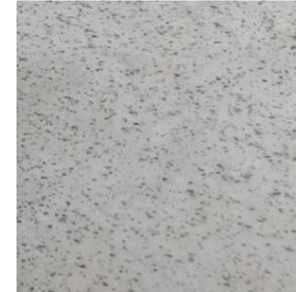
SALT FINISH CONCRETE FLOORING
