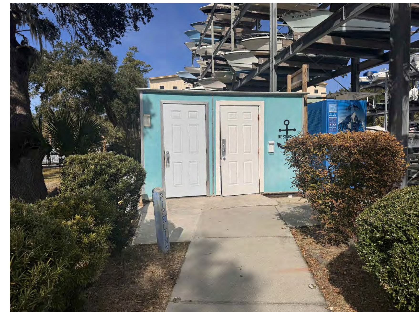
BROAD CREEK MARINA - PUBLIC RESTROOMS
