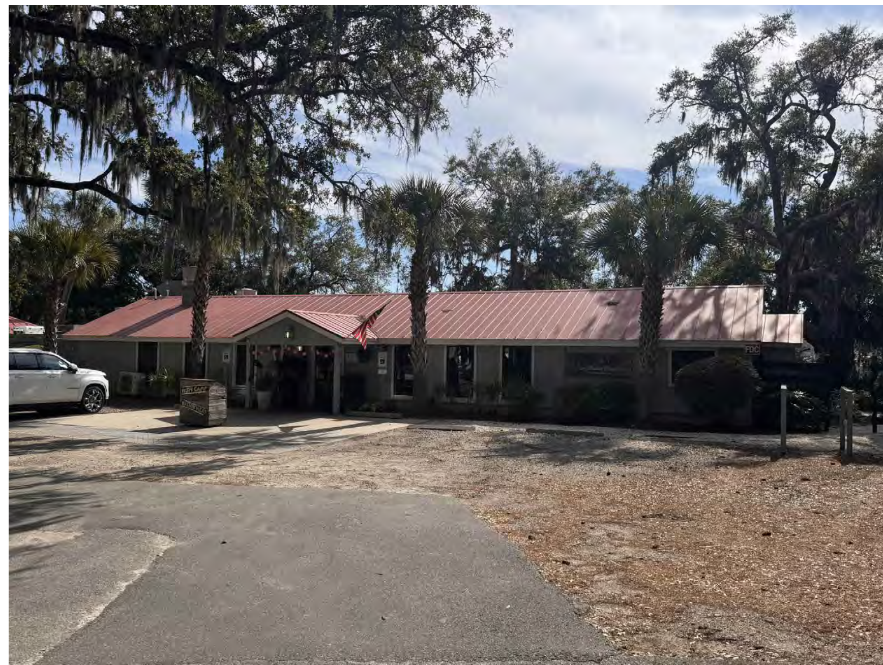
FISH CAMP - ADJACENT STRUCTURE
