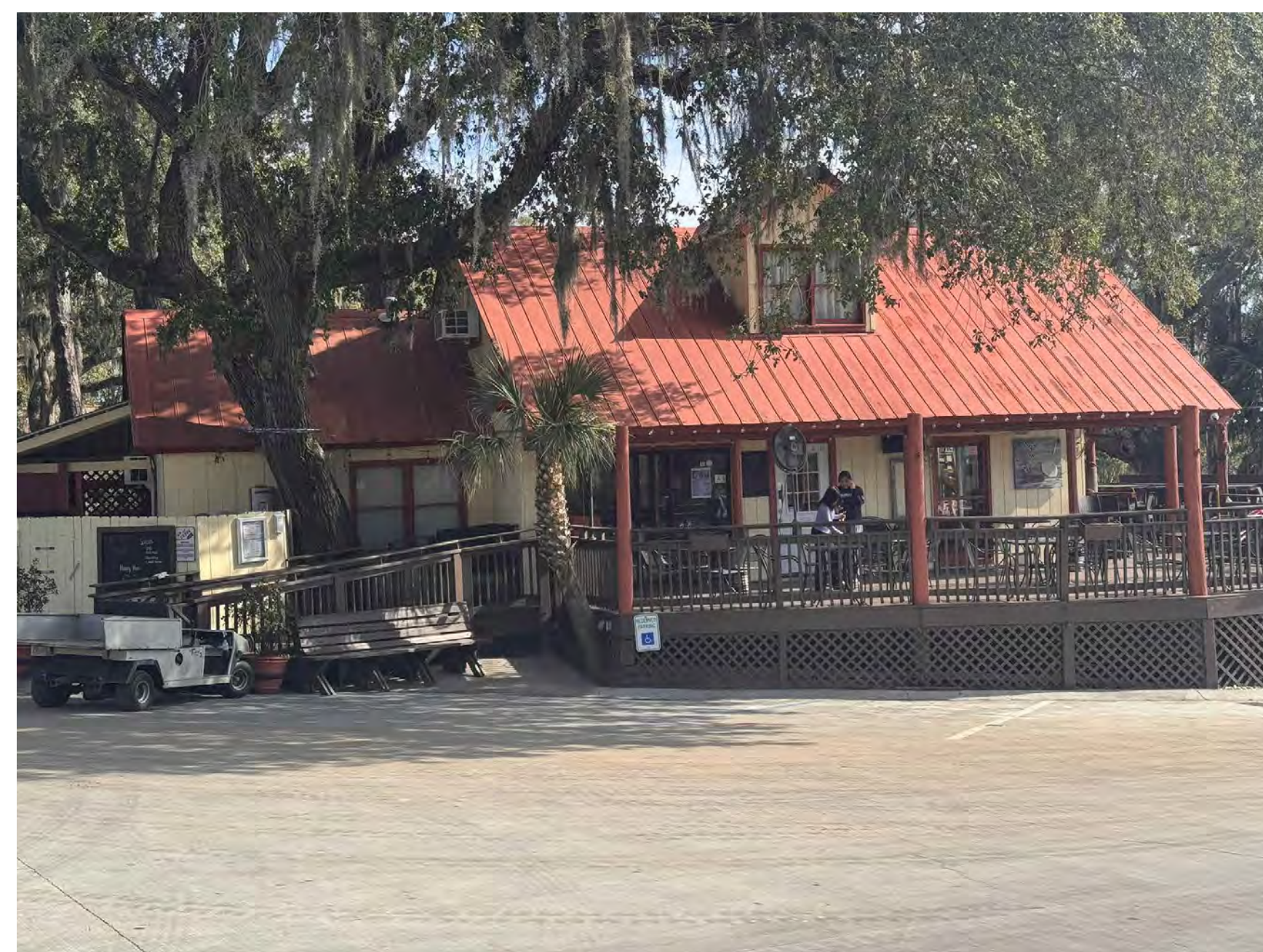
UP DA CREEK - ADJACENT STRUCTURE
