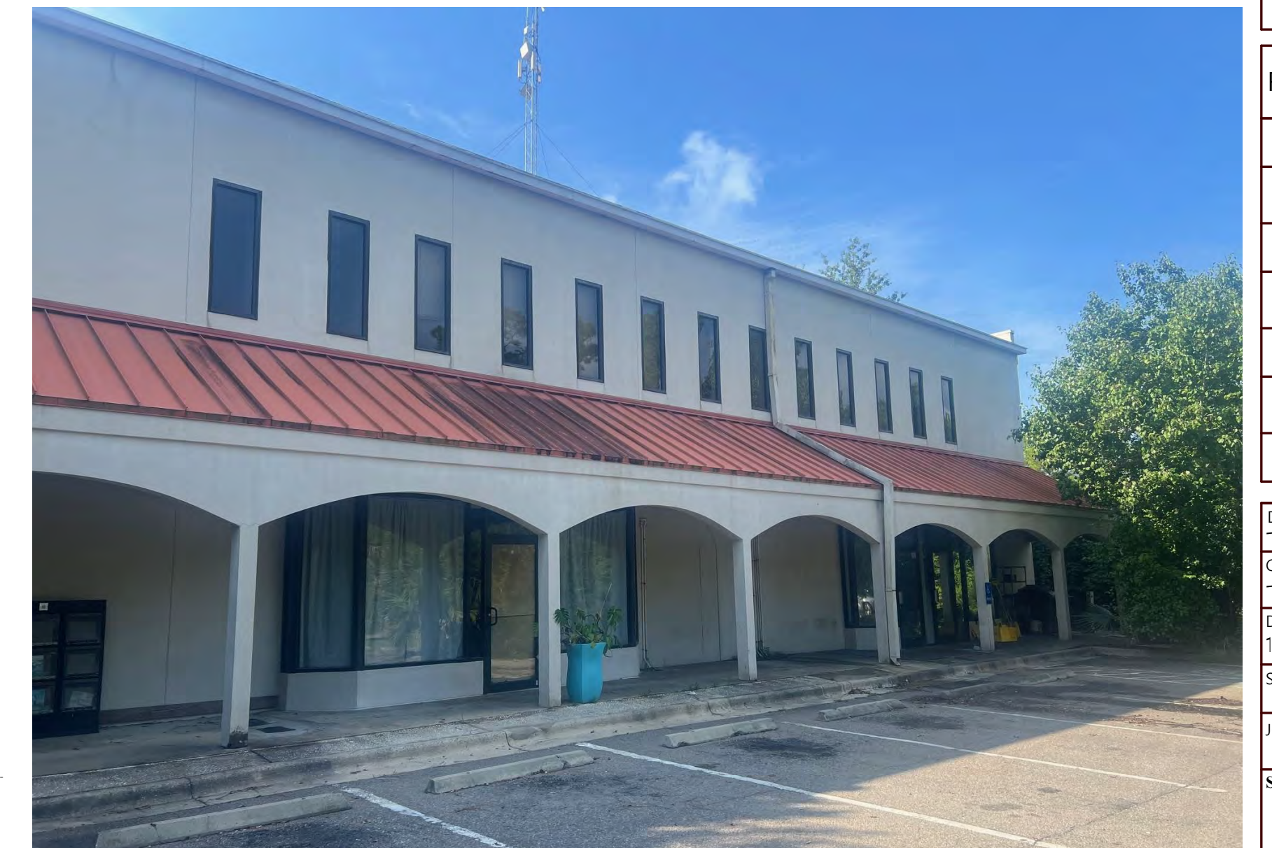
EXISTING RIGHT SIDE ELEVATION PHOTOS
