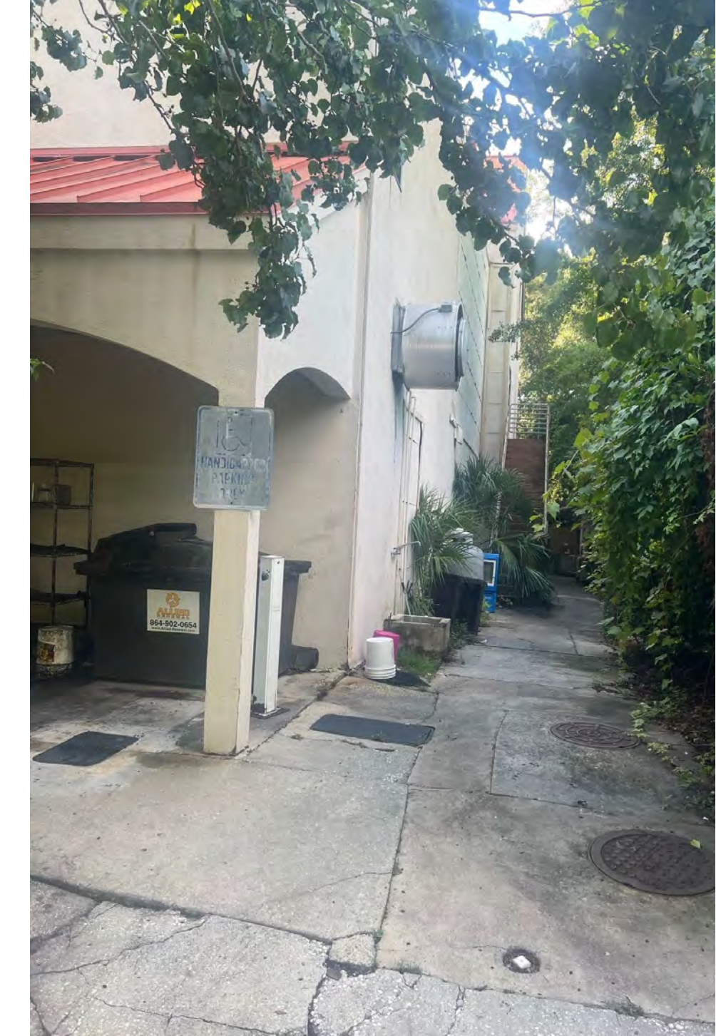
EXISTING REAR PHOTOS
