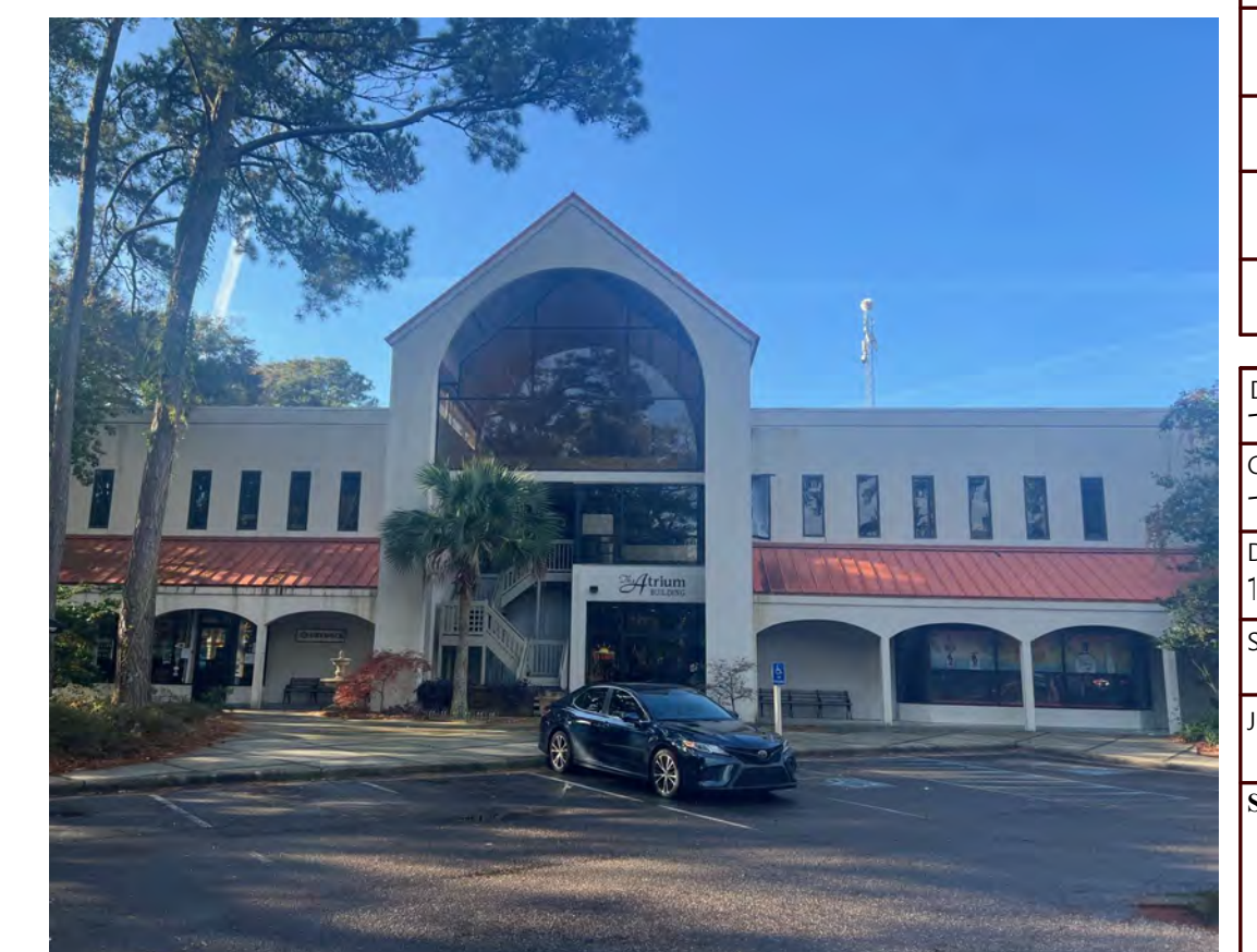
EXISTING ENTRY PHOTO
