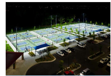
IMAGES ABOVE ILLUSTRATE DIRECTIONALITY OF LIGHT THROW TOWARDS PICKLEBALL COURTS NOTE: LIGHT POLES ON OUR SITE ARE 25'
