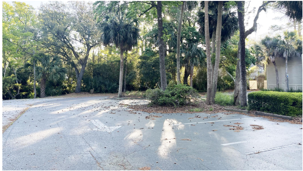
ASPHALT PARKING LOT
