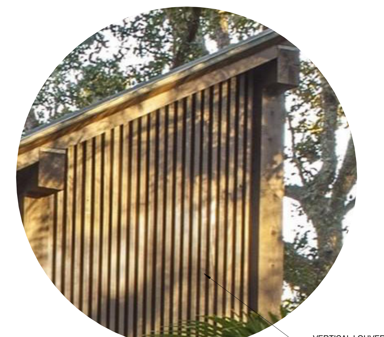
EXAMPLE OF VERTICAL LOUVERS SHOWN FOR REFERENCE.
