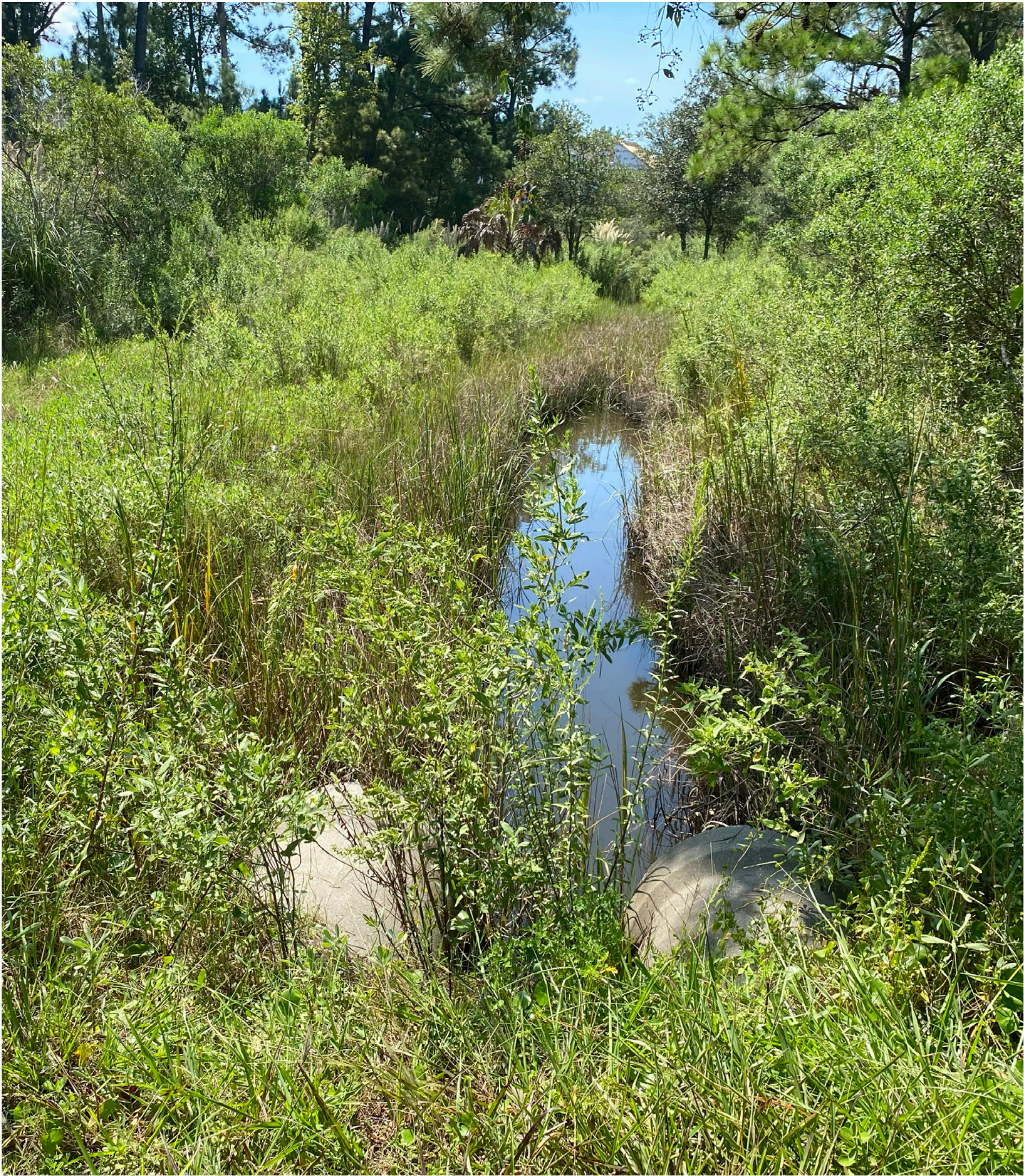
EXISTING STORMWATER DITCH
