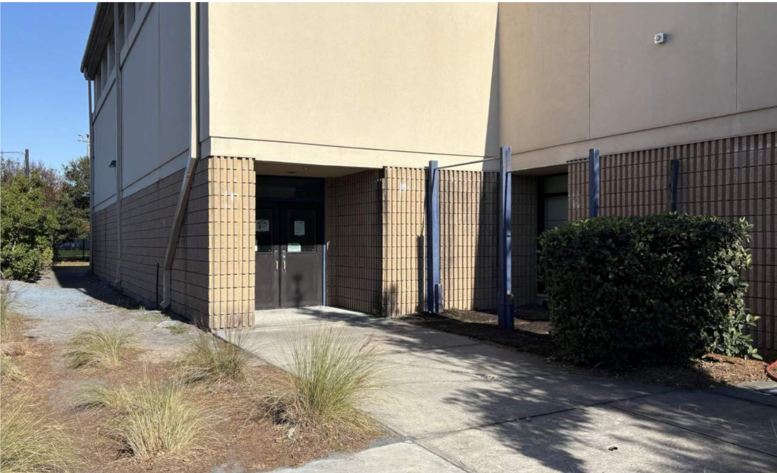
EXISTING SOUTH - AUXILIARY GYM ENTRY
