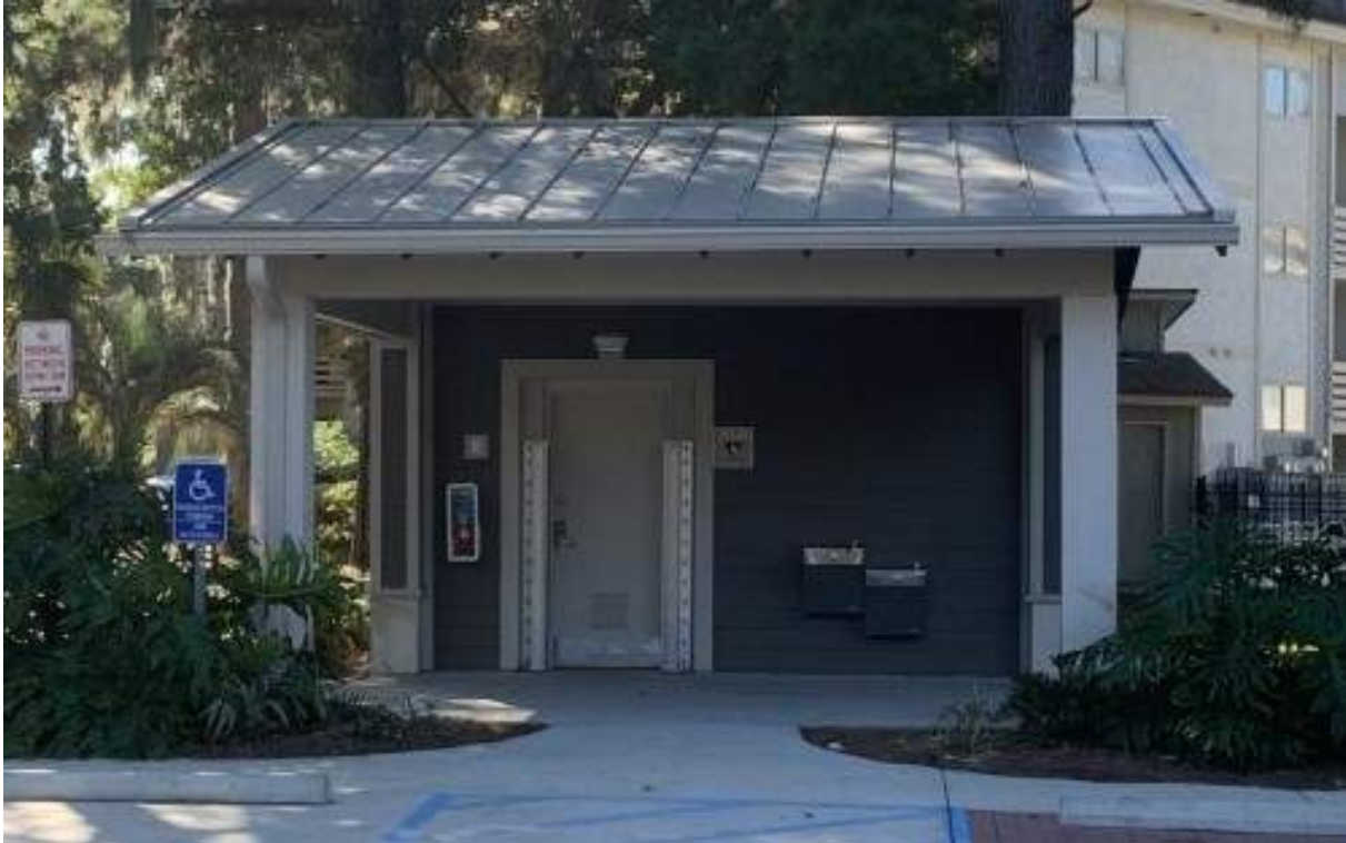
View of existing facility on Cordillo Parkway that new building will match.
