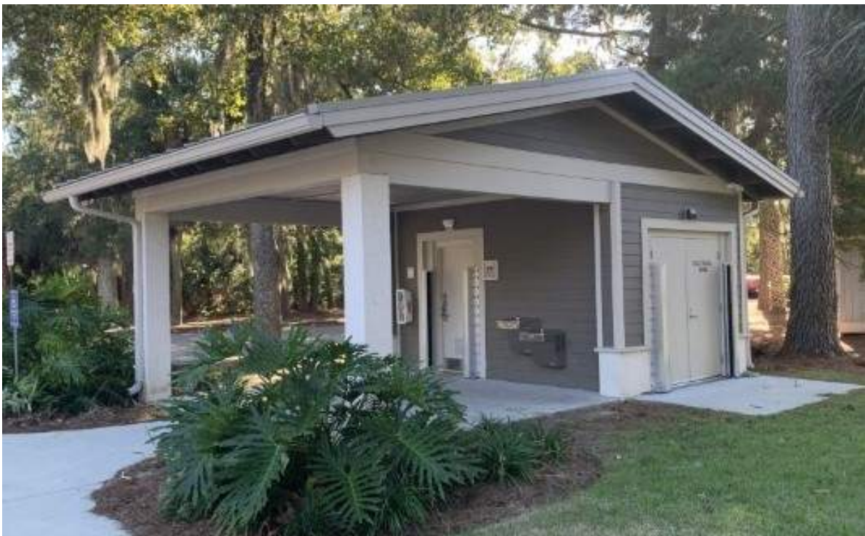
View of existing facility on Cordillo Parkway that new building will match.
