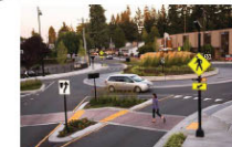
2B RFB WARNING MARKINGS AND SIGN
